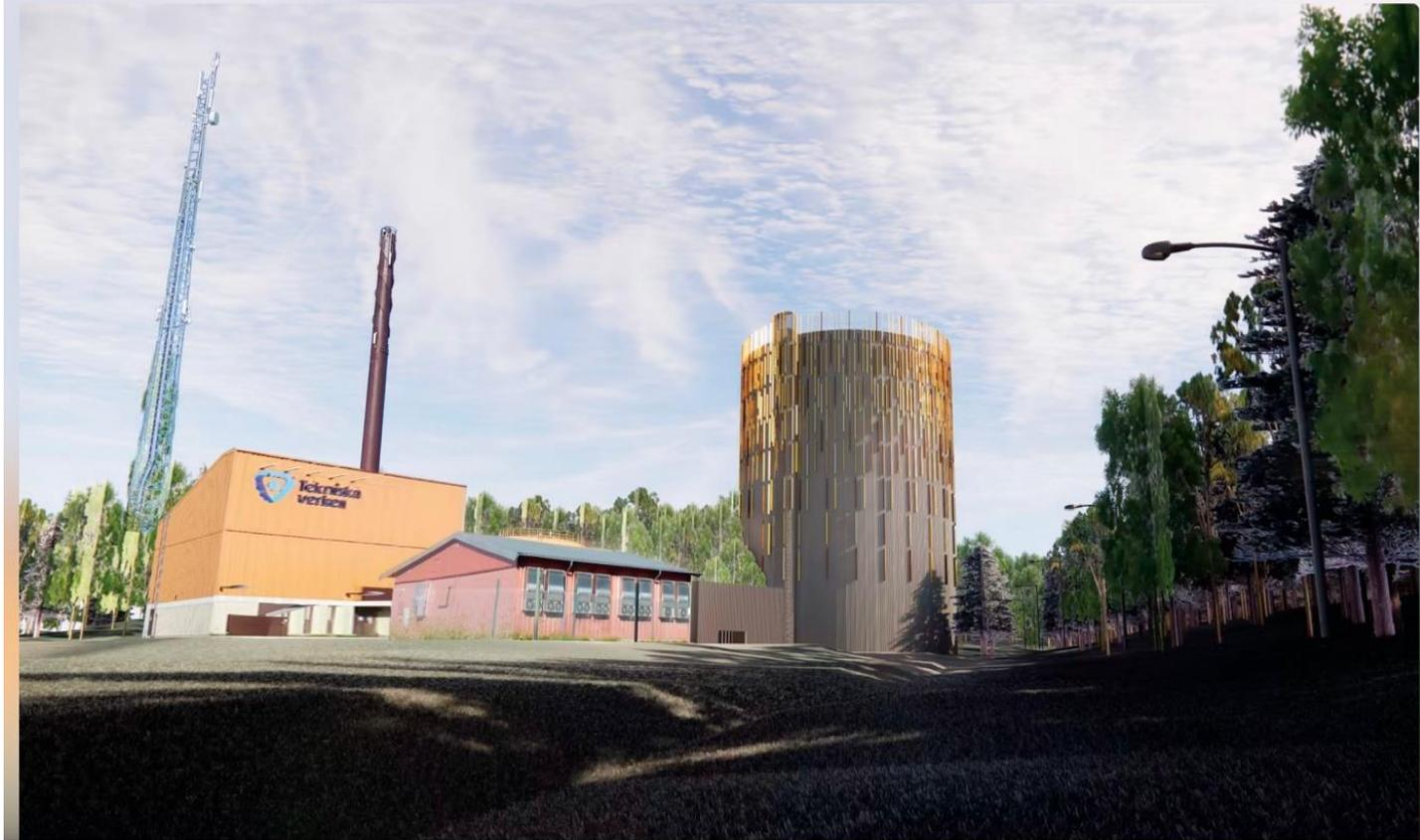
*New hot water accumulator in Linköping. The accumulator will have an energy capacity of 1.4 GWh. It holds 30 000 m<sup>3</sup> water. It has an inner diameter of 33 meters, and is 45 meters high. The in-load capacity is 40 MW and the out-load capacity 60 MW, with a maximum temperature of 98°C.*
