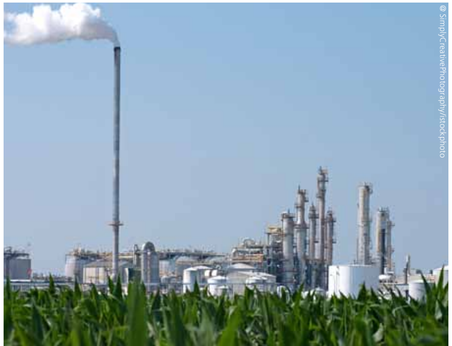
Ethanol plant by corn field.
