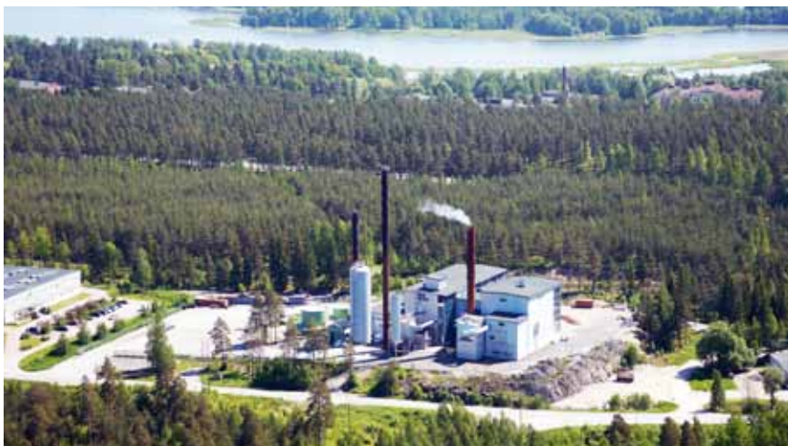
Ekenäs Energi in Finland is a bioenergy CHP with the capacity of 17 MW thermal and 3,4 MW electricity. Photo: KMW Energi
