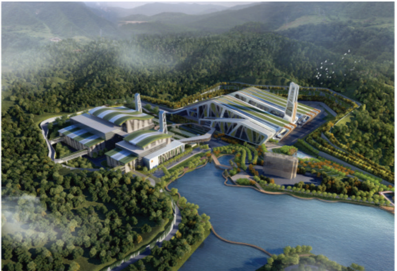
Facility in Shenzhen, China. Phase III Baoan WtE is built with Keppel Seghers technology. The plant will process waste equivalent to 46 truckloads every hour, or 9000 tonnes per day. The energy produced is enough for 3 million citizens or 13 million 40W light bulbs. This will replace the generating capacity of 700 000 tonnes of coal each year, with the effect of cutting CO 2 emissions by around 2 million tonnes per year.
